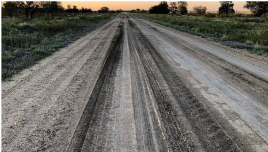
Figure 14: Boo Boo Road north of Gurley Station entrance -deformation due to lack of gravel and widened road as vehicles avoid centre of road
