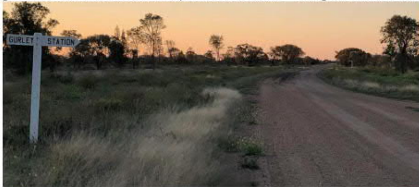
Figure 14: Boo Boo Road north of Gurley Station entrance -deformation due to lack of gravel and widened road as vehicles avoid centre of road
