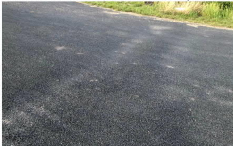
Figure 17: Minor road deformation over culvert at Boo Boo-Gurley Creek road intersection
